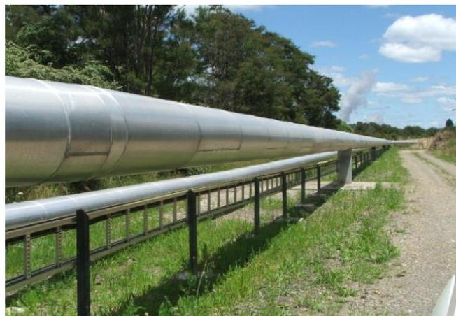
*Pipelines all run about one to two metres above the ground and are held on support structures concreted into the ground.*
